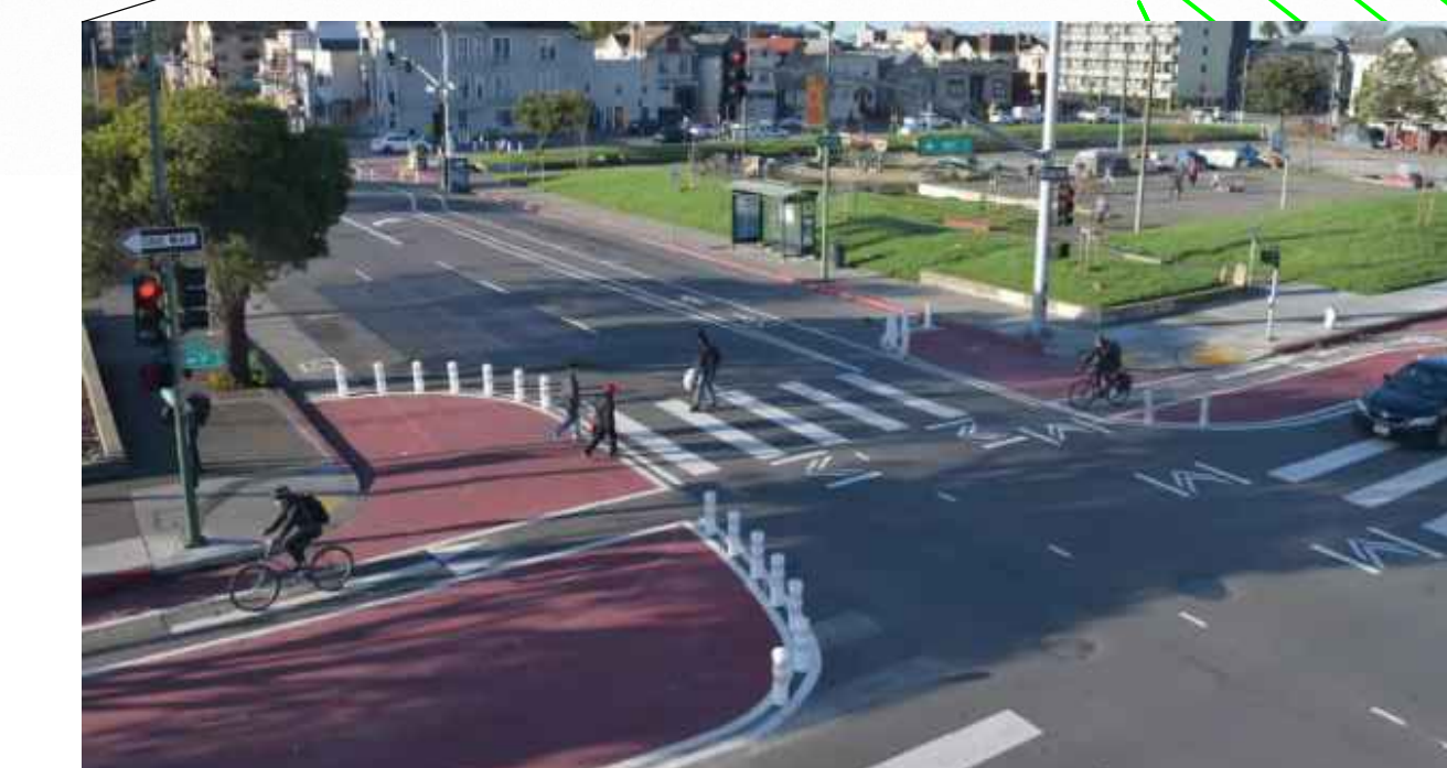
QUICK-BUILD PROTECTED INTERSECTION
